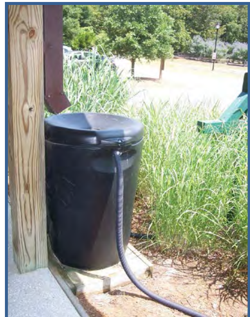
Figure H-8 Typical rain barrel adjacent to a flower garden. (Photo courtesy of Daniel Newquist, Waccamaw Regional COG)
