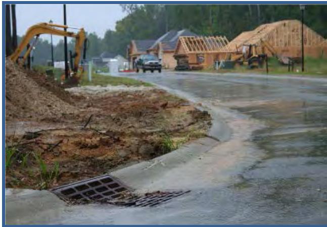
Figures G-2 and G-3 Construction site activities that disturb soil can cause sedimentation problems in nearby waterways. Storm drain protection devices shown on the right can help prevent downstream water quality problems. (Photos courtesy of Horry County Stormwater Department and US EPA.)
