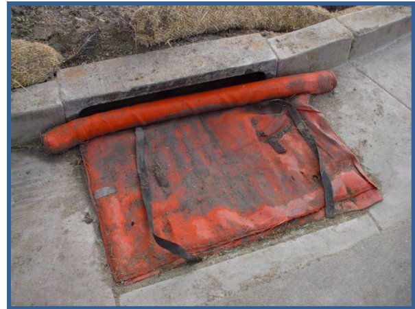
Figures G-2 and G-3 Construction site activities that disturb soil can cause sedimentation problems in nearby waterways. Storm drain protection devices shown on the right can help prevent downstream water quality problems. (Photos courtesy of Horry County Stormwater Department and US EPA.)
