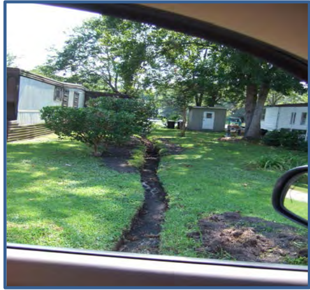
Figures C-11 and C-12: The stormwater infrastructure system within the watershed consists of an extensive network of canals, ditches, ponds, pipes, and outfalls. In some cases, residents have attempted to address localized drainage issues by constructing small scale ditches. These practices can exacerbate erosion problems and potentially affect drainage patterns in downstream areas nearby. (Photos Courtesy of Dan Newquist, Waccamaw Regional COG and Dr. Dan Hitchcock, Clemson University)
